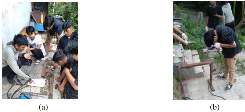
Figure 4. (a) Group discussion analyze project design (b) Welding process
